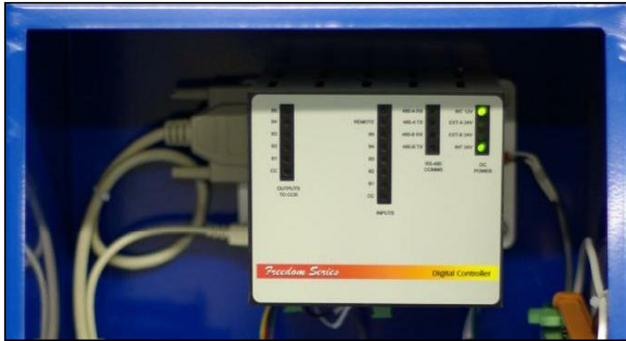
Fig. 3 DCMU adds L-827 Monitoring and IRMS capability to existing CCRs and a redundant RS485 Modbus communications interface to a new 3rd party ALCMS.
