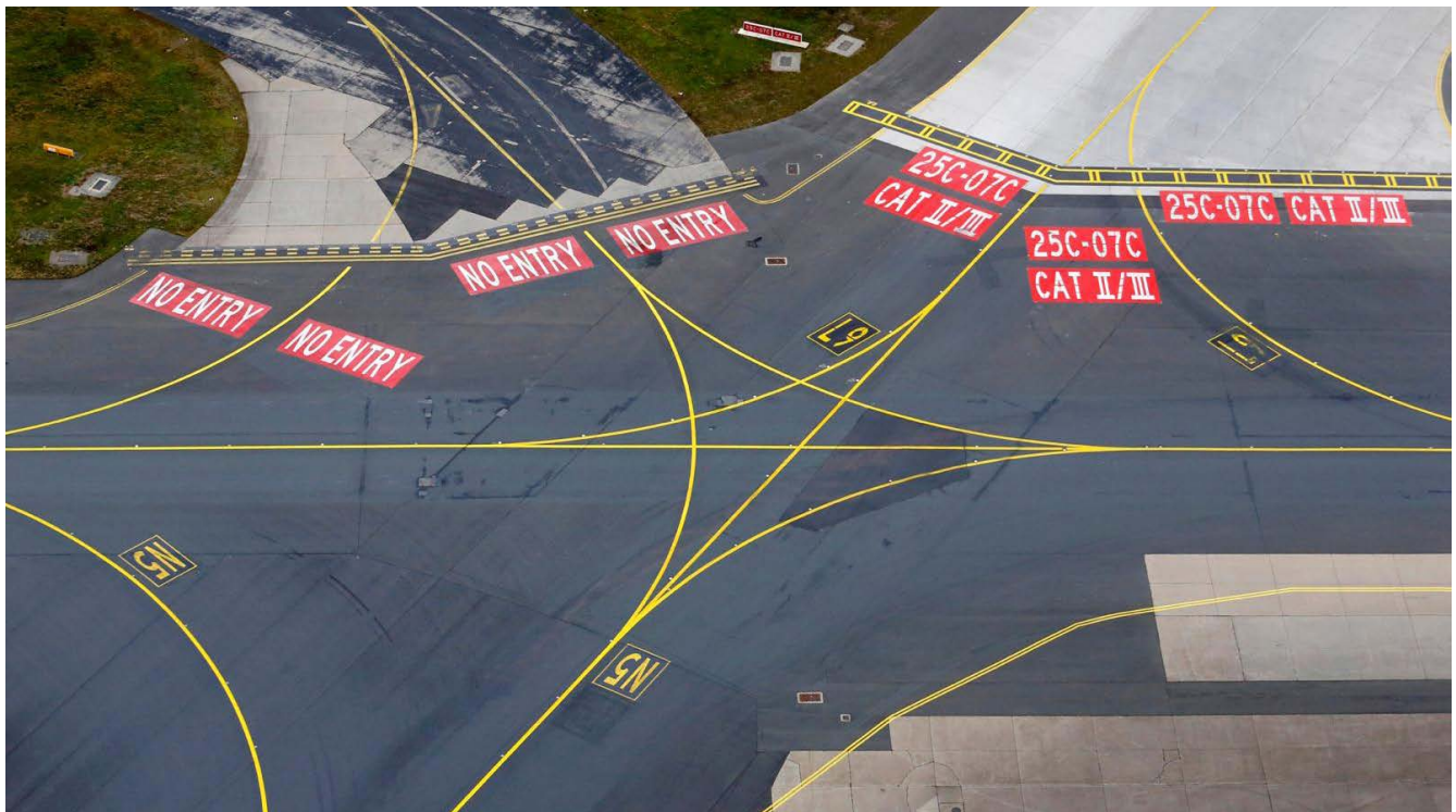
▲ Figure 13 – Markings and signage at CAT II/III Holding Position at Frankfurt Airport (Source: Fraport AG)
